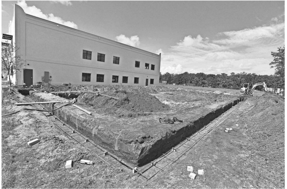
A trench is prepared for the footers of what will be the Jacksonville University Satellite Campus building in the initial Fountains development area. The buildout of the Fountains St. Johns development project off County Road 210 near I-95 in northern Saint Johns continues with retail, office space and residential housing all underway on July 14. BOB SELF/FLORIDA TIMES-UNION
